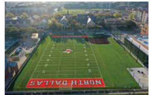
Photo provided by Paragon Sports Constructors-North Dallas HS.
