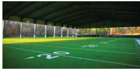
Photos provided by Hellas Construction-Marshall ISD
